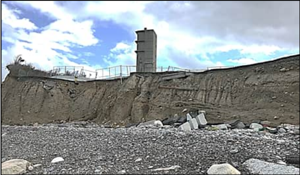
Exhibit 1: Existing Cliff Debris (Taken November 2021)
