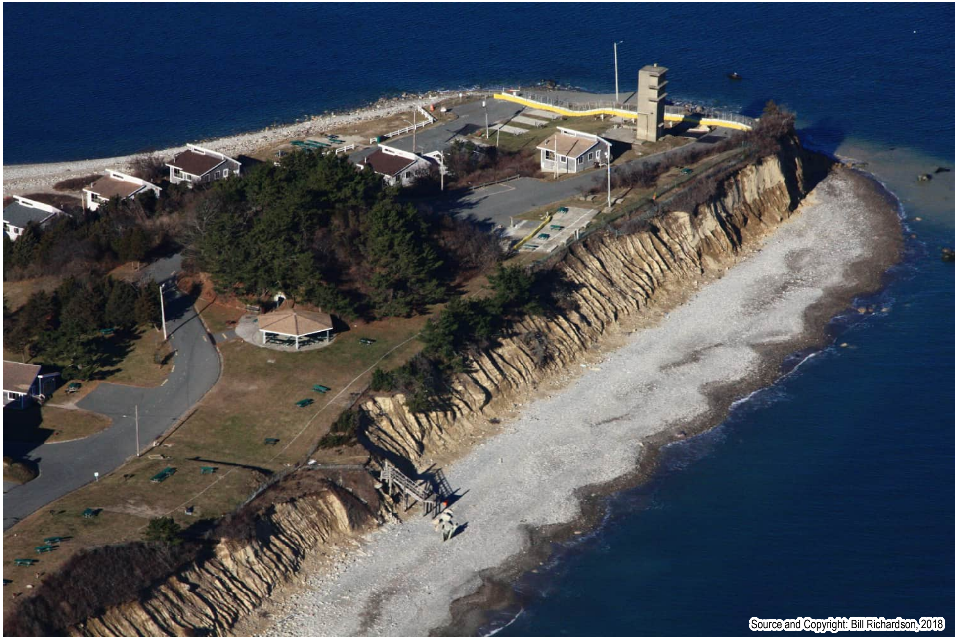
Figure 1-5: Fourth Cliff Existing Conditions-East Bank Closeup
