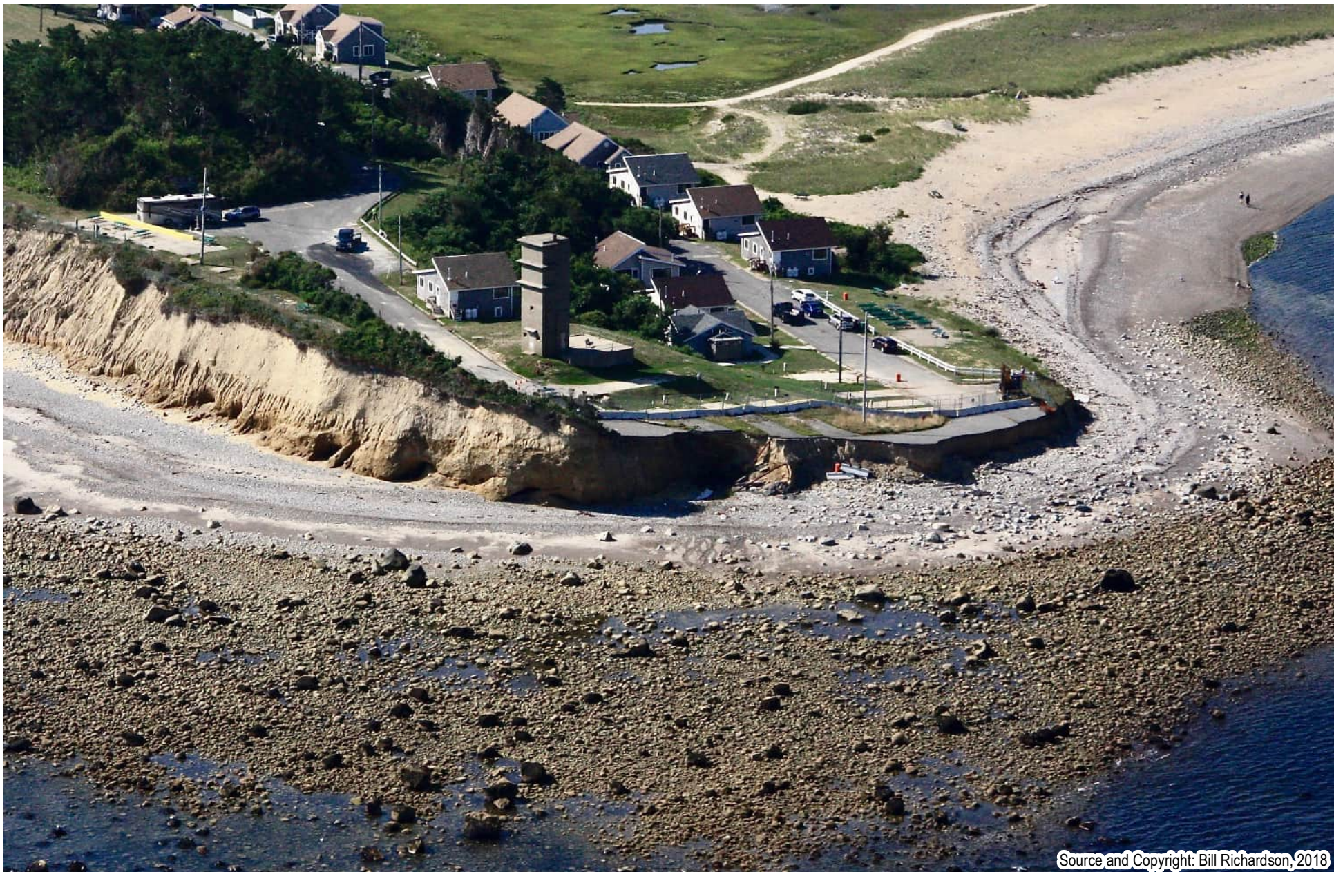
Figure 1-2: Fourth Cliff Existing Conditions-Toe
